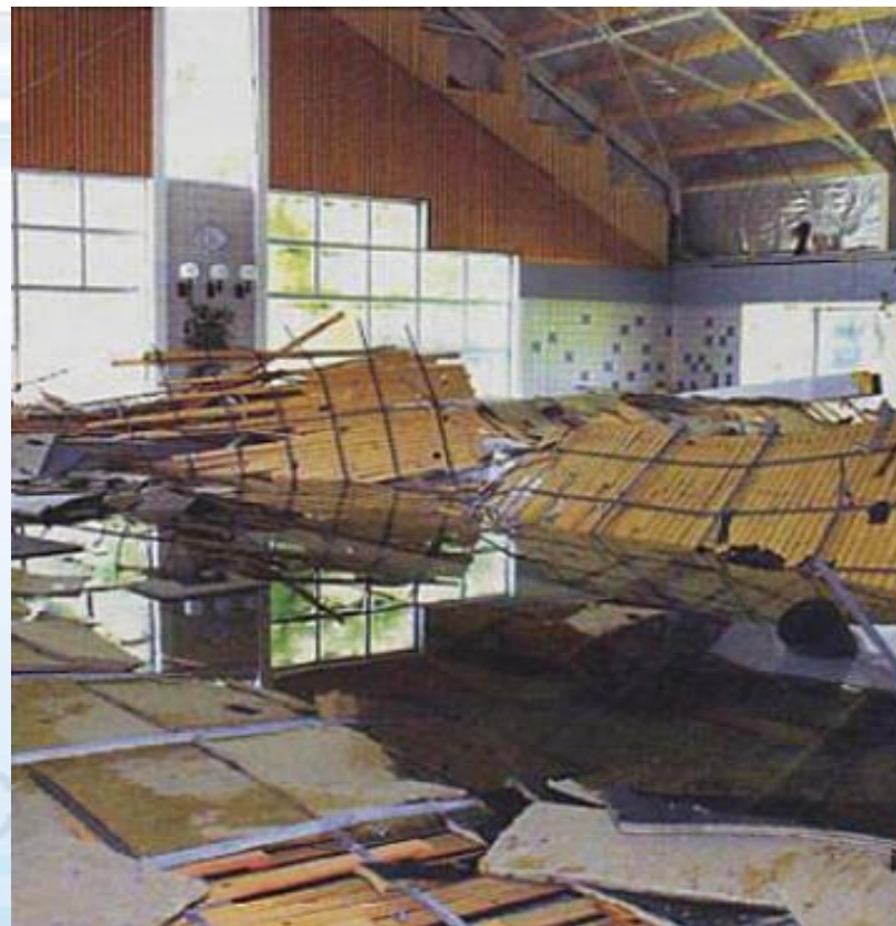
Ceiling collapse in The Netherlands
